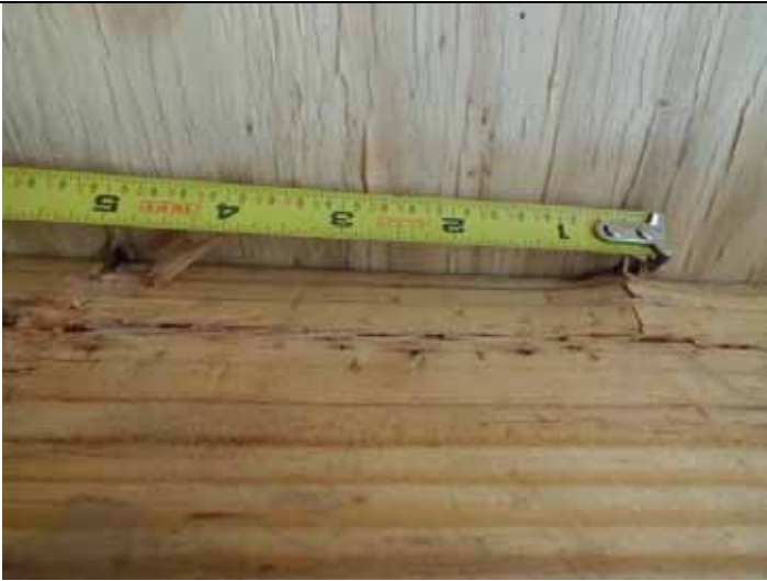
Roof deck attachment
