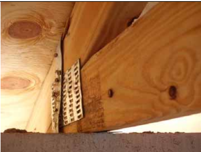
Roof to wall attachment
