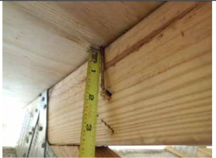
Roof deck attachment
